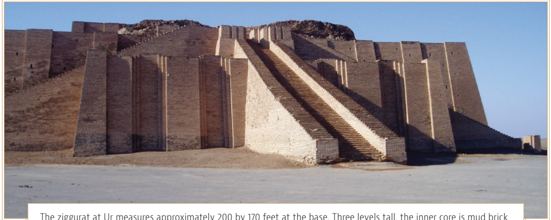
The ziggurat at Ur measures approximately 200 by 170 feet at the base. Three levels tall, the inner core is mud brick while the outer shell, which is 8 feet thick, is baked brick. At the top was a temple to Nanna, the moon god.
